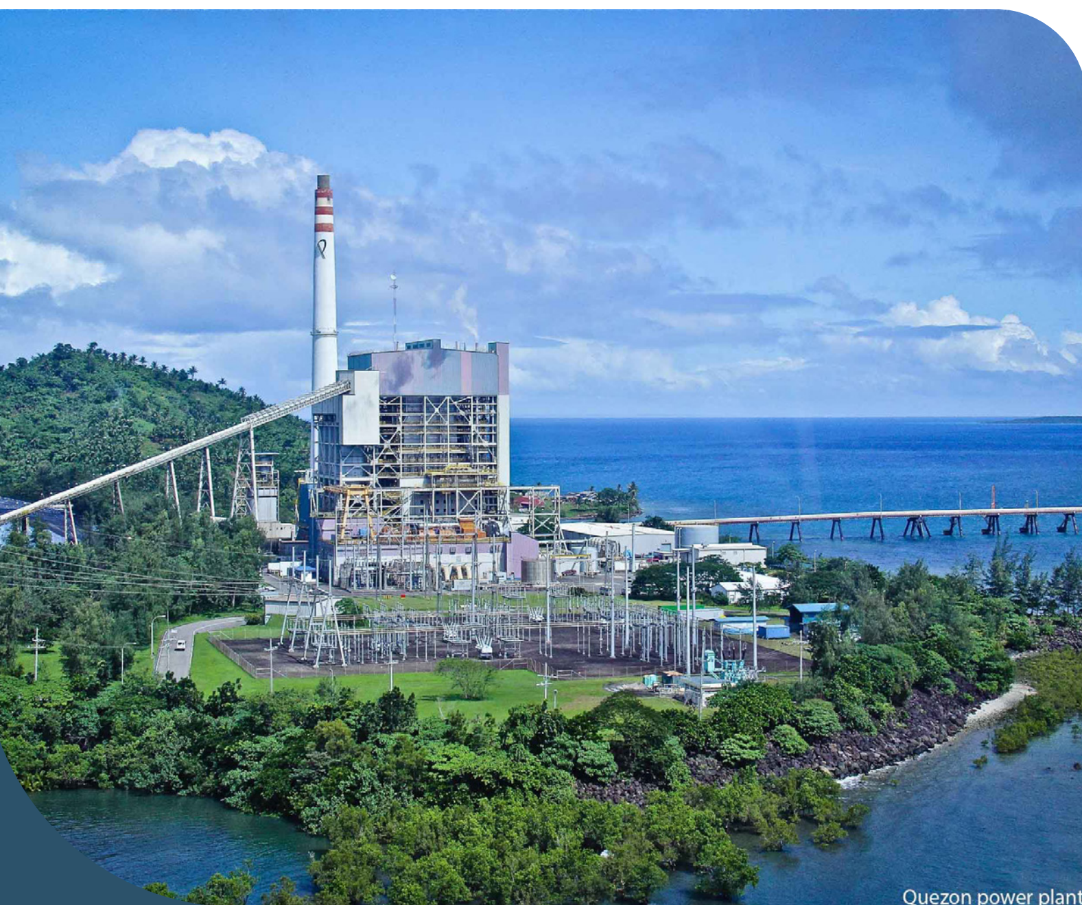
Quezon power plant
